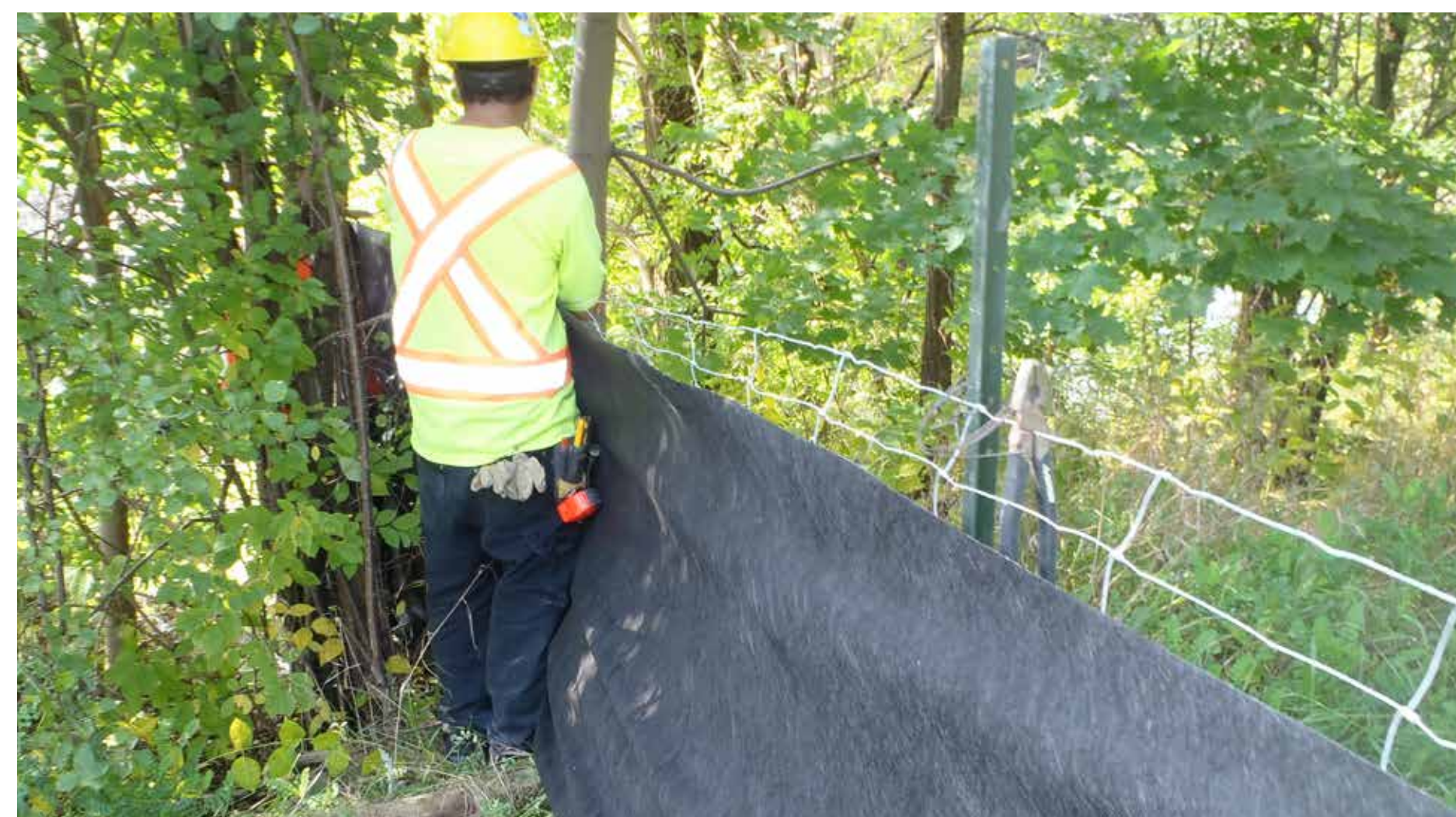
Example of sediment control fence being installed
